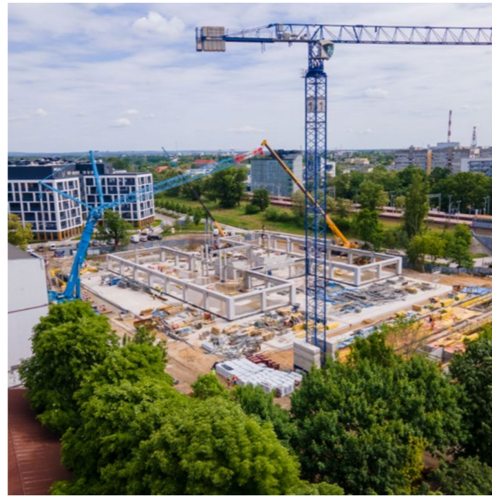
Element Hotel construction site, Wroclaw, Poland
